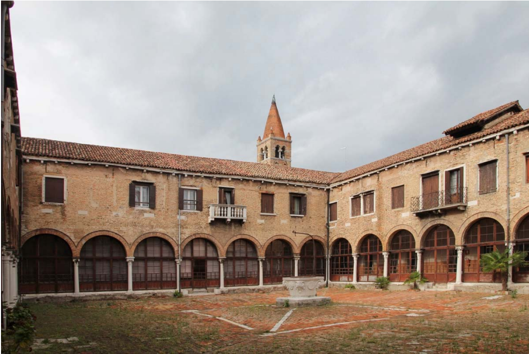
Campo S. Alvise, Istituto Figlie della Carità Canossiane: Empty complex of houses with potential for housing inhabitants (Bernhard Furrer, October 2015)
