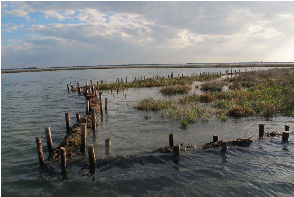
The "industrial" recreation of lost saltmarshes ( barene ) by depositing sediments dredged elsewhere in the Lagoon (as part of the MoSE construction works) is showing promising results: regrowth of saltmarsh vegetation; nevertheless the lost ecosystem is not yet recovered and it may still take substantial time until a full restoration of the saltmarshes. (Tobias Salathé, October 2015)
