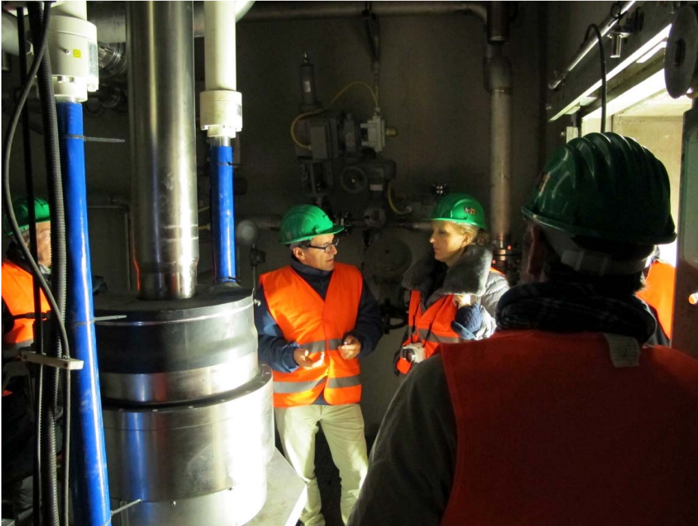
UNESCO mission at the hydraulic pumps of the MoSE system underneath the Lido Lagoon inlet. (Tobias Salathé, October 2015)
